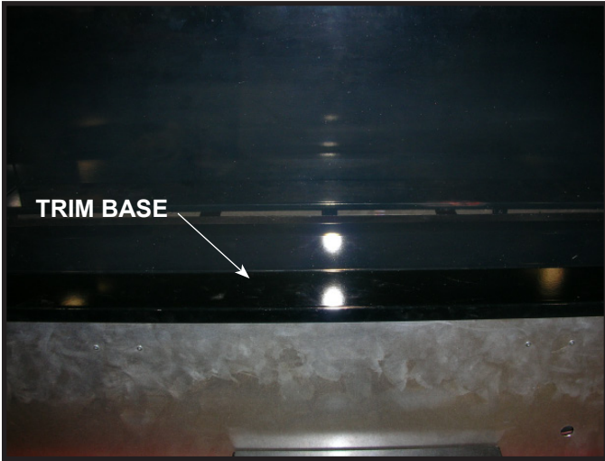
Figure 14. Porcelain Trim Base Installed.
